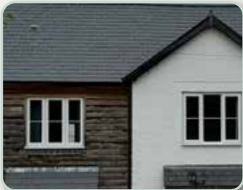
Natural timber weatherboarding, lightly rendered brick
