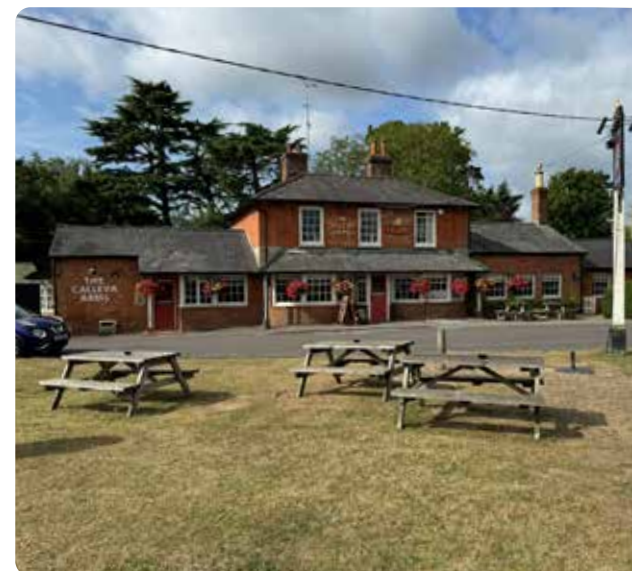
Figure 23: The Calleva Arms features a tiled hipped roof with smaller scaled catslide overhang roofs at the front and defining white frame windows spanning the façade.
