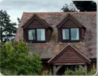
Gable dormers and porch with timber weatherboarding
