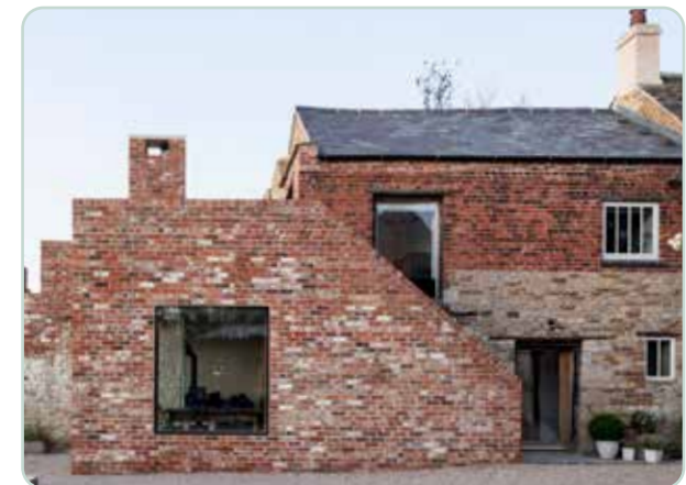
Figure 72: Recycled and reclaimed bricks used for an extension to a traditional dwelling in Gretton, UK. Image credit: Johan Dehlin, Source: https://www.archdaily.com/
